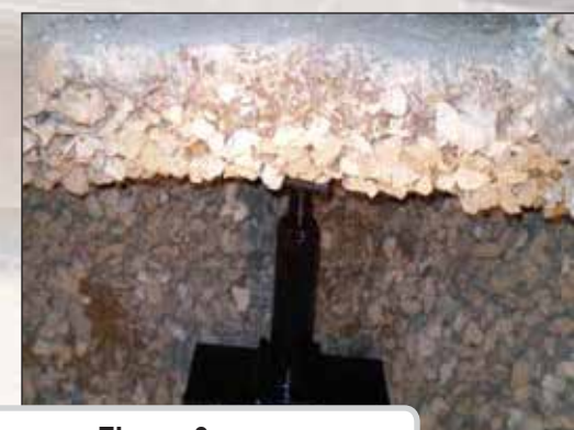
Figure 3 Structure is now carefully lifted, or stabilized to eliminate further settlement
